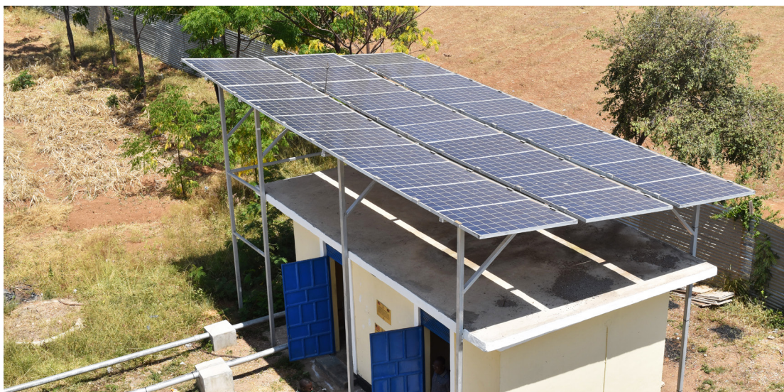
Solar panels installation
